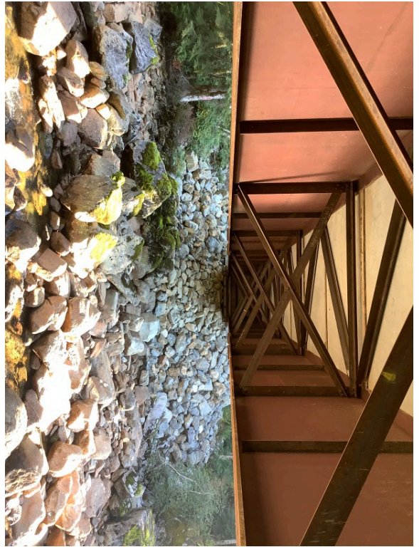
Left Bank Abutment when facing downstream
