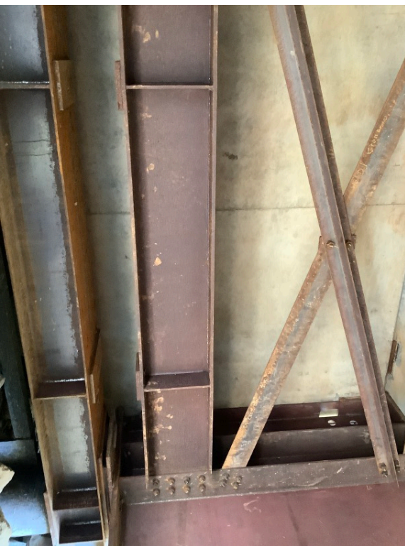
Right Bank Abutment when facing downstream
